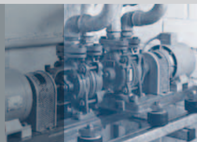
AOH pumps for water distribution in domestic applications.
